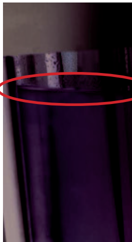
Dust and dirt particles in the refrigerant. Visual inspection to determine the degree of fouling.
